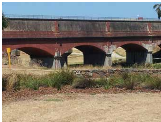
Historic Sewage out fall Bridge along the Federation Trail
